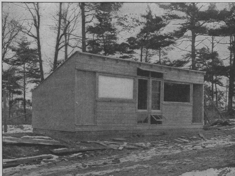
FIG. 8.— The Cornell poultry house with pens 12 feet square. There is a door in the partition between pens. The cloth curtain is made of loosely woven unbleached muslin
