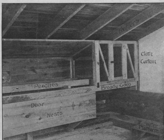
FIG. 12.— The broody coop, nests, and roosting fixtures in the Cornell poultry house with pens 12 feet square
